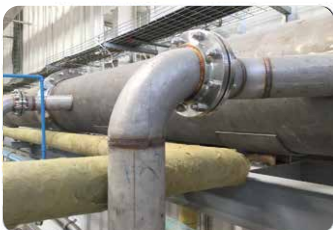
SS Piping Work
